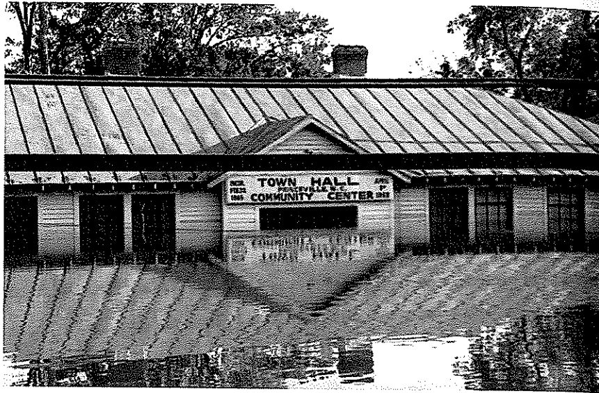
Princeville's old town hall mostly submerged in the floodwaters of Hurricane Floyd, 1999. Photo Credit: The Town of Princeville, NC.
